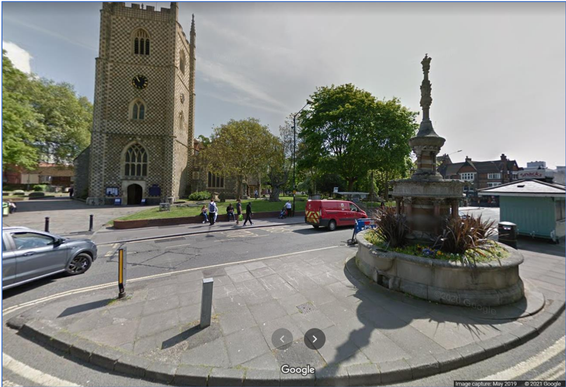
View of the application site from corner of Hoiser Street and St Mary's Butts. Google Street view image captured in May 2019.
