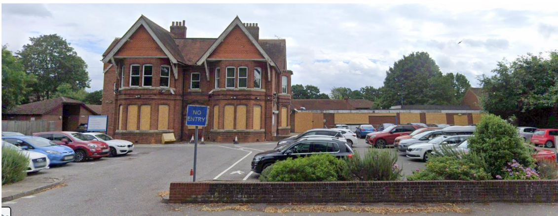
View of Hospital building from Liebenrood Road
