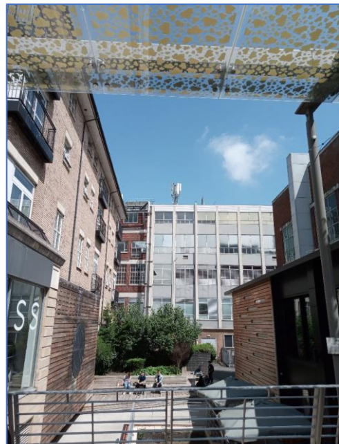
Fig 4. Existing rooftop equipment to 41 Minster Street as viewed from the walkway from Gun Street/Minster Street to The Oracle Shopping Centre.
